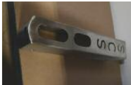
Pivot protectors strengthen, protect, and repair, timber double-swing doors.
